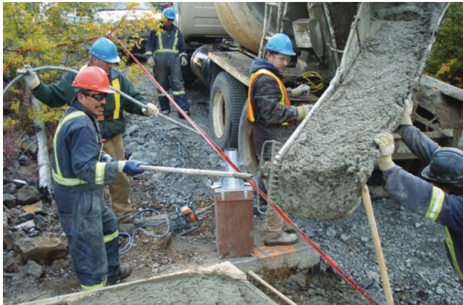
Figure 11. Pouring concrete to cap a mine opening, Port Radium, 2007. Published in Indian and Northern Affairs Canada, “How has the Port Radium Remediation Project made the site safer for people, animals, and the environment?” Winter 2009. Photo courtesy of the Délı̄nę Knowledge Centre.
