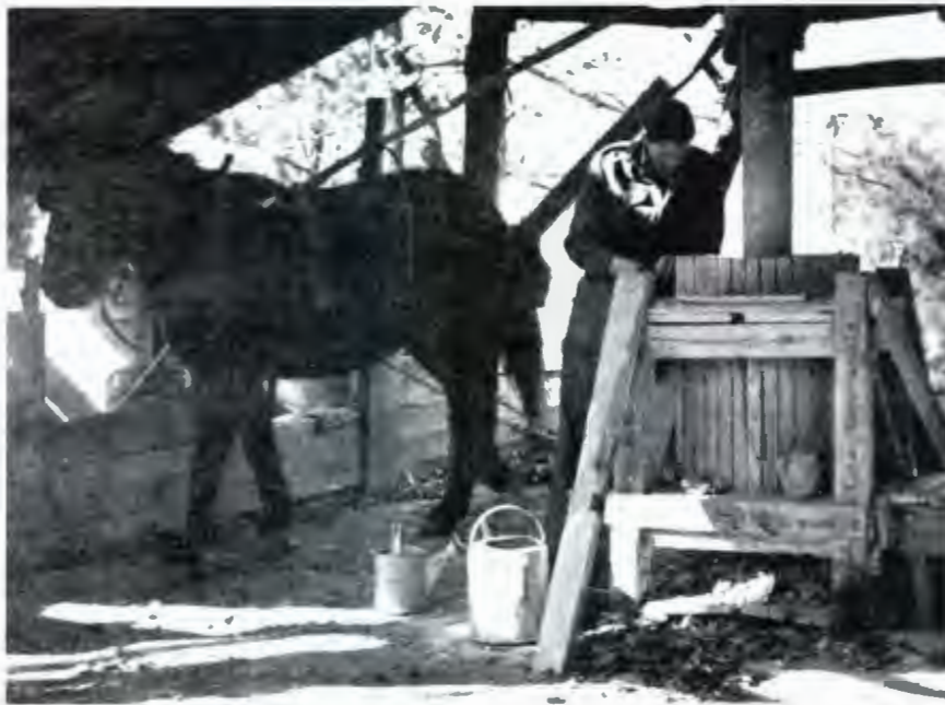
Figure 11: Grinding clay with a horse powered pug mill (Webster 1971: 44).
