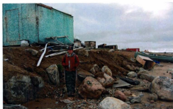
Figure 3.55 View looking east along the shoreline. Coastal erosion is occurring along this portion of Patricia Bay. Boulders were placed to armour the slope against wave erosion, however sediment loss is still occurring (photo T. Bell, July 2007).
