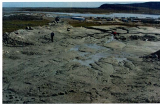
Figure 3.64 Most infrastructure in Clyde River is built on pads constructed using sand and silt. Sand is not a suitable material for construction as it is very easily eroded (photo M. Irvine, July 2007).
