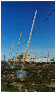
Figure 3.46 Leaning telephone poles in Clyde River illustrate differential settling and ground movement (photo M. Irvine, July 2007).
