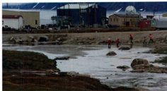
Figure 3.43 View looking southwest at children playing in the main stream that runs through the community. Water is accumulating on the upstream end of this culvert because it has been infilled by sediment and debris. Ground thaw in front of the culvert has lowered the ground surface below the bottom of the culvert, necessitating a lowering of the culvert in order to make it function properly (photo M. Irvine, July 2007).
