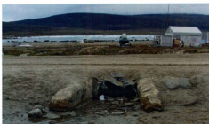
Figure 3.68 View looking south towards Patricia Bay. This culvert currently drains water from the southeast part of town into the beach area. If sea levels rise, during storm events or storm surges, sea water could flow back through this culvert, and others under the road, causing flooding in the lower portions of the community (photo M. Irvine, July 2009).
