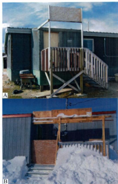
Figure 3.40 Local infrastructure adaptations (photos M. Irvine, July 2007 and March 2010). A) In Clyde River wind scoops are built in front of doorways to direct drifting snow away from the door. B) The effectiveness of the wind scoop varies, and will depend on factors such as the height and distance of the wind scoop from the doorway and the wind direction.
