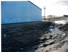
Figure 3.56 View looking west at one end of the arena (grey building). Erosion and slumping are occurring along the stream bordering the foundation pad of the Clyde River arena and sports complex. The sediment in this area, which is similar to that underlying much of Clyde River, consists of easily erodible marine sand and silt (photo M. Irvine, July 2007).
