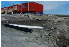
Figure 3.65 Houses in Clyde River are built on silty-sand pads. After rain events, sediment is washed downslope, and expensive remediation efforts are required. The black and white rolls in the foreground of the photo are geofabric and plastic grid that are used to stabilize the sediment on the slope and under the houses (photo M. Irvine, July 2007).
