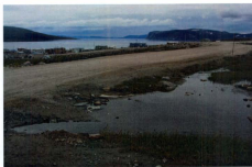
Figure 3.44 View looking southeast from an area of projected development at the mid-slope above town. Water pooling is occurring along the side of the road because there is no culvert in place to drain it (photo M. Irvine, August 2008).
