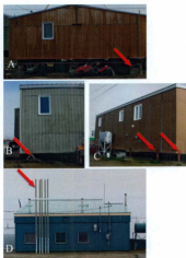
Figure 2.2 Examples of building foundation-types found in Clyde River. A) a house built on cribbing; B) a house with jacks; C) a house with steel piles; and D) building employing thermosiphons (photos M. Irvine, July and August 2007).
