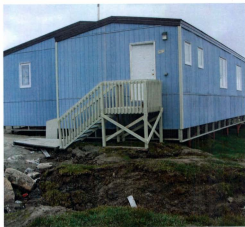
Figure 3.57 Thermal erosion and resultant settling of ice-rich permafrost is causing damage to the porch of a house in the centre of Clyde River (photo M. Irvine, July 2007).
