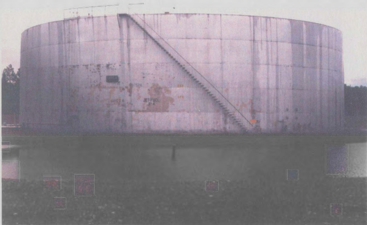
Figure 1.3: Photograph of Upper Tank Farm (UTF) storage facility (12 million litres, Jet Fuel - JP4) located on top of south escarpment.
