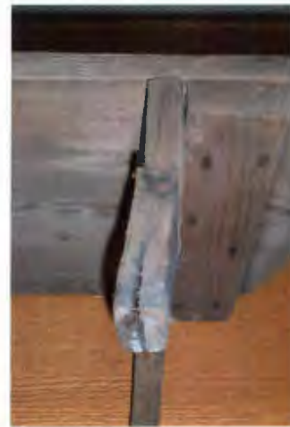
Fig. 7) Detail of rotted and badly-patched milking stool leg. NMSTC 2001-0232.
