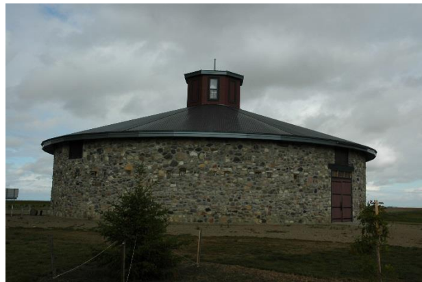
Figure 45: The rebuilt Bell Barn is an example of a rare barn type in Saskatchewan: the round barn, constructed of local fieldstone. Indian Head. September 1, 2013.
