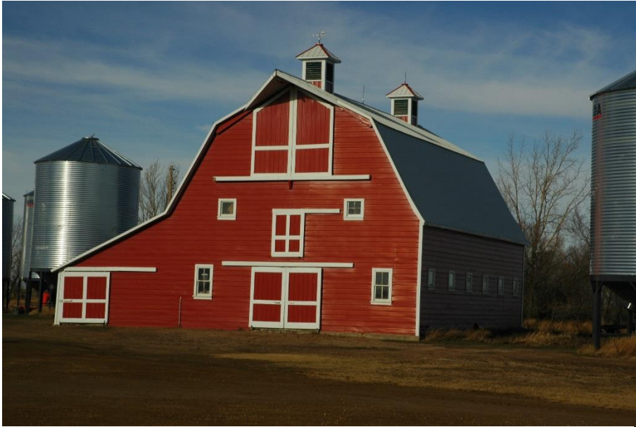
Figure 37: The Verot barn has been clad in red tin on the south side; the north side awaits the same treatment. The R.M. of Laurier No. 38, southeast of Radville. November 15, 2013.
