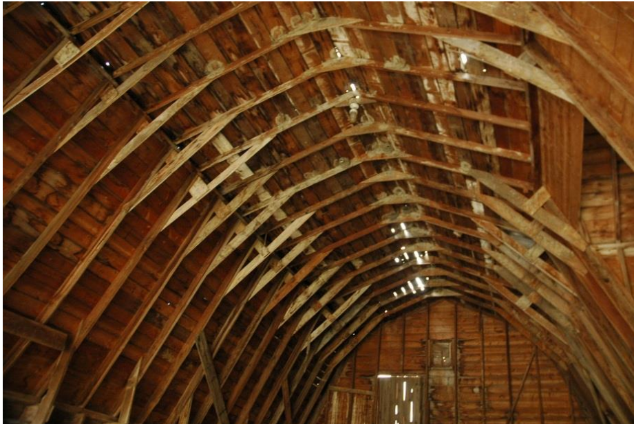
Figure 17: The exposed trusses of a gambrel-roofed barn displays the plank- framing construction method that was exclusively used in my study region. R.M. of the Gap, east of Ceylon. September 9, 2013.
