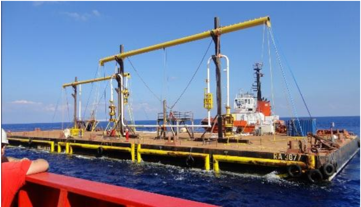
Figure 9 Offshore Transportation Of The Rigged Spool.
