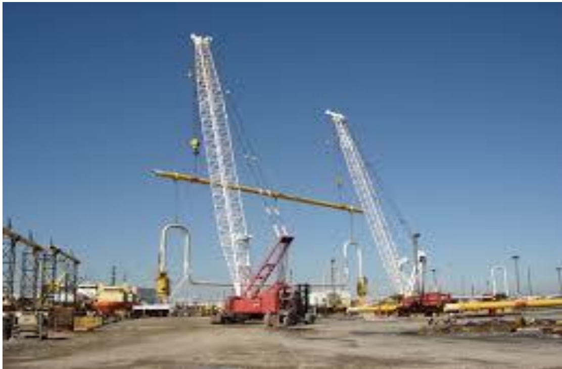
Figure 8 Land Transportation of Rigged Spool
