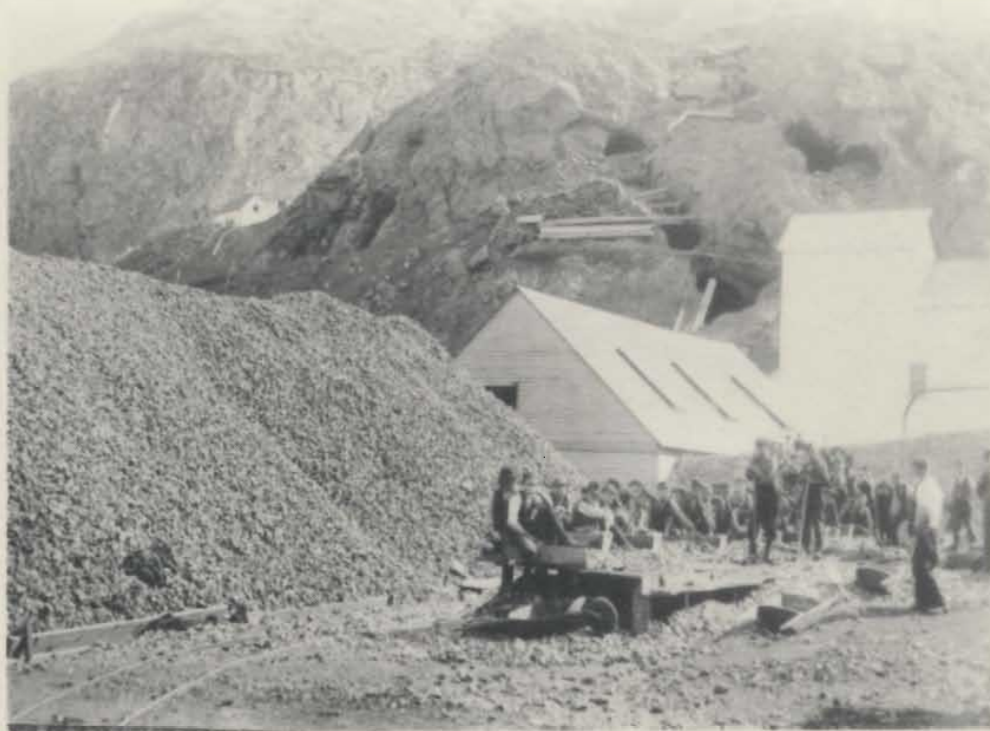
Figure 2. An early mining operation in Newfoundland. Note the track for hauling the ore from the mine and the hand tools being used. Similar tools were used in building the railway beds of Newfoundland railways.
