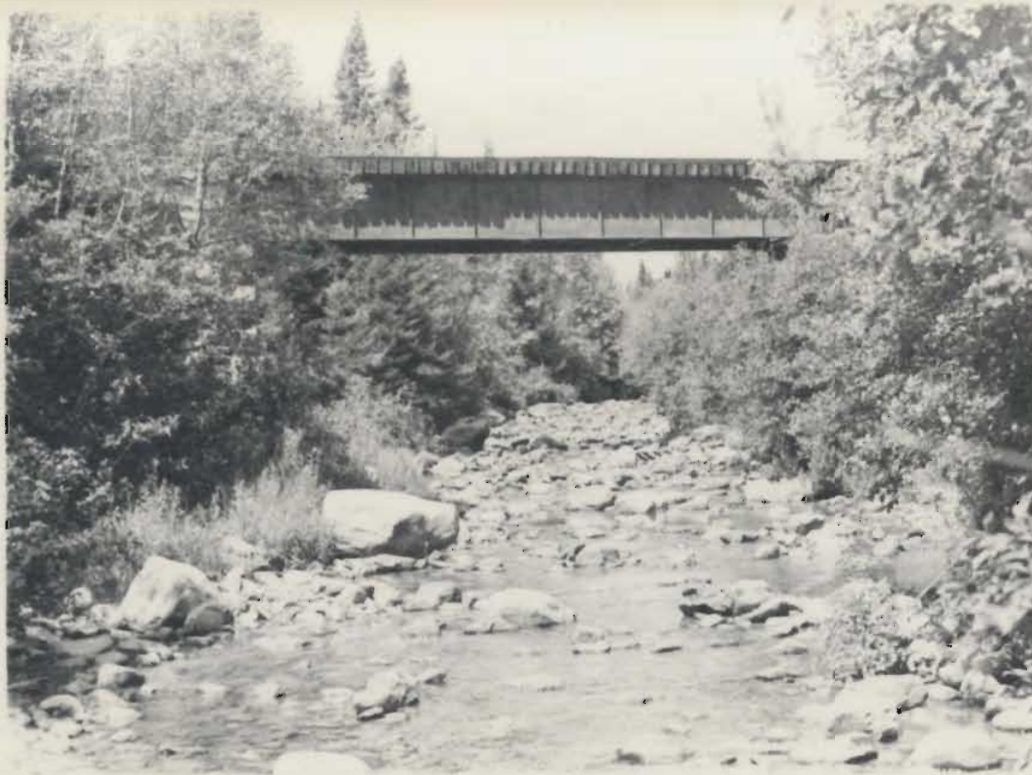
Figure 17. Dark Hole Bridge, near Clarendville (lower Shoal Harbour). This bridge -- built by Reid -- was typical of the many railway bridges required to span the numerous small streams and their valleys which the railway followed and crossed on its route across the Island. Dark Hole River was diverted from its original river bed a short distance east to Lower Shoal Harbour River so that its waters would not undermine the railroad bed.
