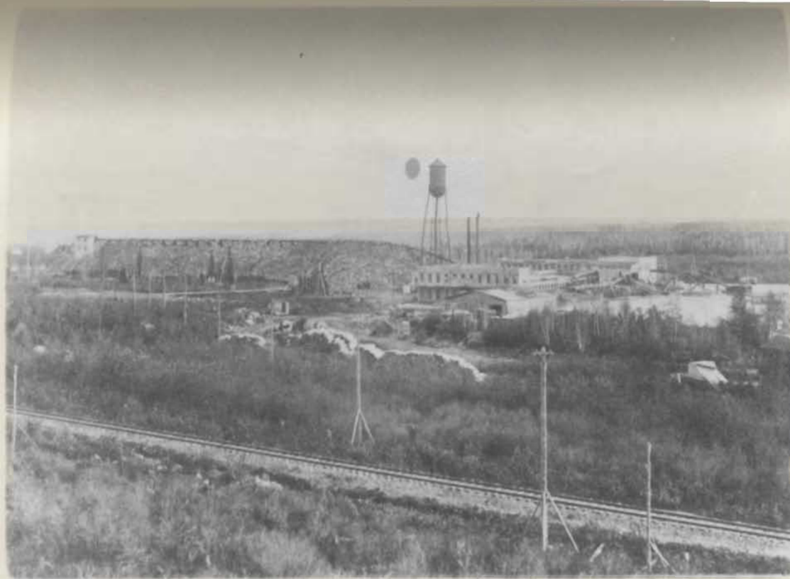
Figure 51. Pulp mill at Bishop's Falls; part of the pulp and paper operations of the A.N.D. Co. at Bishop's Falls -- Grand Falls. The pulp manufactured here was sent to Grand Falls by a flume to be processed further and made into paper.
