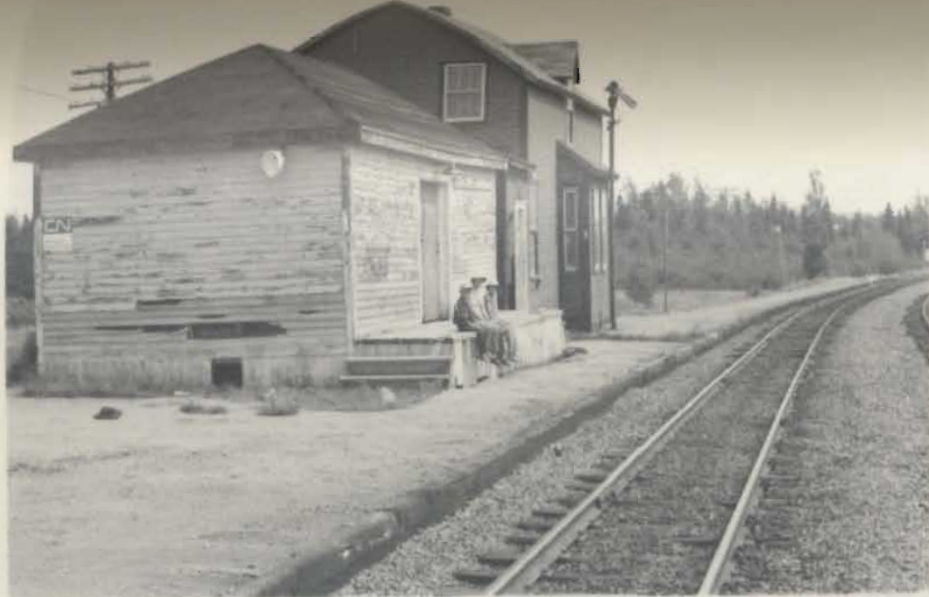
Figure 34. Station House, Notre Dame Junction
