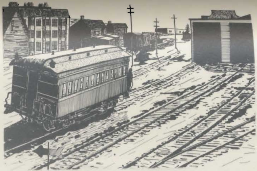
Figure 27. St. John's Station at Fort William (East End, St. John's)
