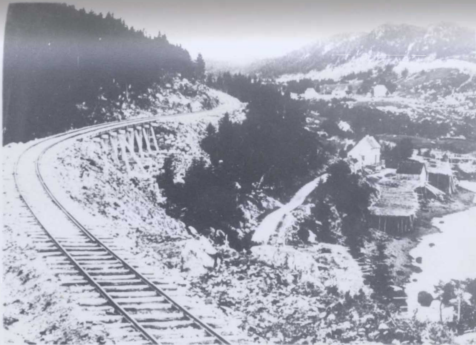
Figure 12. North Arm, Holyrood. From North Arm the railway turned inland towards Harbour Grace Junction (Whitbourne). Shown here is a dry trestle (later replaced by a retaining wall and earth fill) which enabled the railway to negotiate the steep walls of the hills overlooking a small road and the sea below.
