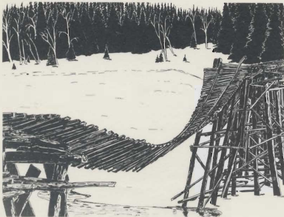
Figure 20. The first trestle built across the Exploits River was destroyed in 1895 by the annual spring break-up of river ice. A permanent structure was built as quickly as possible next to it during the early Spring and Summer of 1895.
