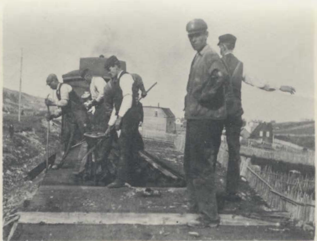
Figure 33. Work train unloading rails, Conception Bay
