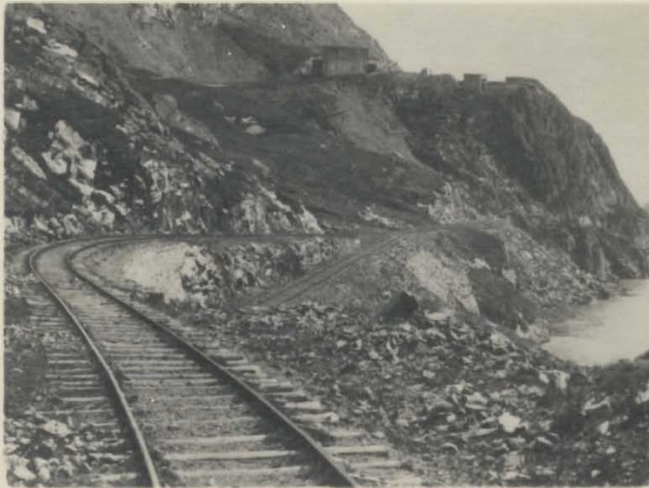
Figure 3. The East End, St. John's Harbour. Note switchbacks shown here (and the steep grades) required so that the railway could descend to the waterfront and a railway finger pier jutting out into the Harbour.
