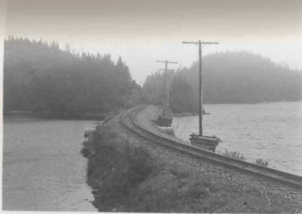
Figure 15. Isthmus of Avalon near Rantem. This was very difficult terrain over which to build a railway solely with the use of hand tools and manual labour. Grades were very steep and many turns, rock cuts, and earth works were required in order to build the railway over the Isthmus of Avalon. Grades were so steep that early steam locomotives could not pull a particularly long or heavily laden train over this stretch of track without first breaking up the train into two sections and making a return trip for the remaining cars.
