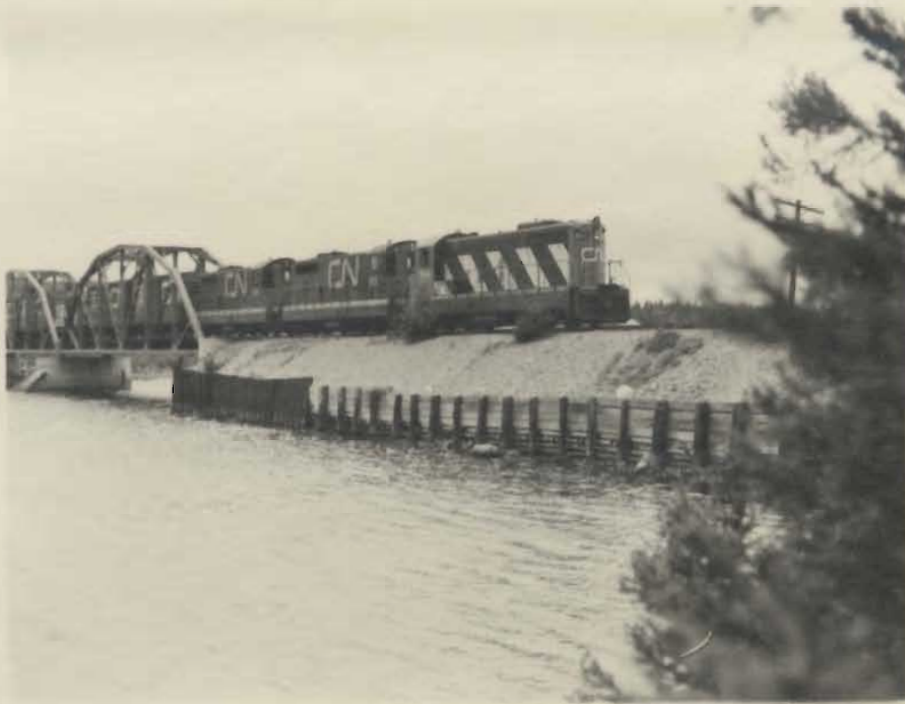
Figure 60. Port Blandford Trestle
