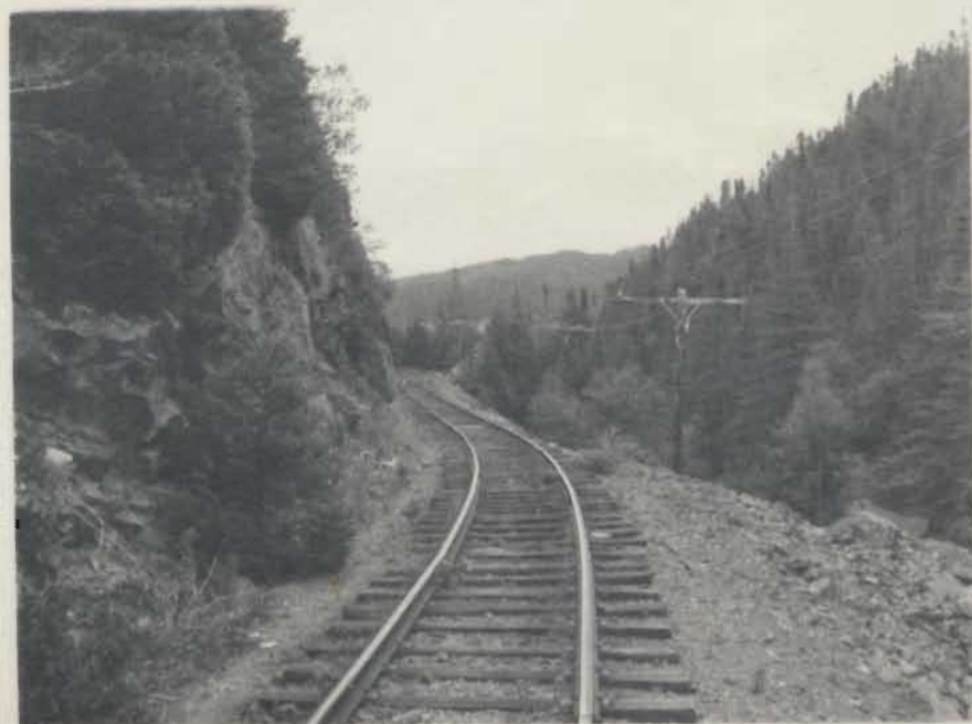
Figure 40. The "Loop" near Goose Cove, Trinity Bay. In order to negotiate the steep incline down to sea level, the railway first passed over an overpass, completely circled a small round pond and then passed under itself and continued down grade through a small river gorge shown in Figure 41 below.
