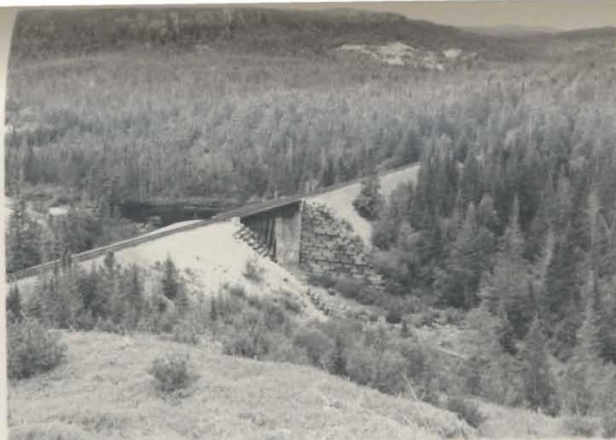
Figure 40. The "Loop" near Goose Cove, Trinity Bay. In order to negotiate the steep incline down to sea level, the railway first passed over an overpass, completely circled a small round pond and then passed under itself and continued down grade through a small river gorge shown in Figure 41 below.
