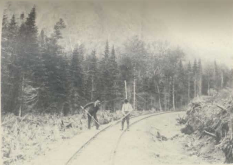
Figure 23. Section men working on the railway near Humber Mouth shortly after the completion of the railway. This short section of track was eventually moved back several hundred yards from the Humber River to make way for a highway which had to share the same route with the railway through a narrow gorge of the Humber River.
