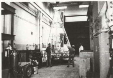
Figure 4.10: Photograph showing the trial matching of the tower supports with the steel base
