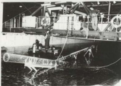
Figure 4.14: Photograph showing the up-ending of the tower in the water near the test location
