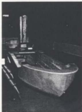
Figure 5.5 M.V. Arctic being ballasted to its design waterline in the ballasting tank. Here, an inclinometer is used to check that the model is not heeled to a significant amount.
