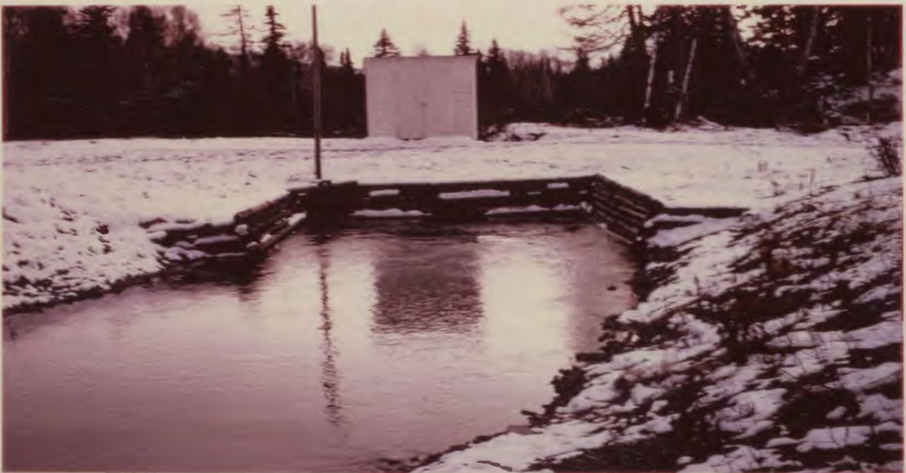
Fig. 7. Water diffuser situated at lower end of water intake structure, Indian River Channel.
