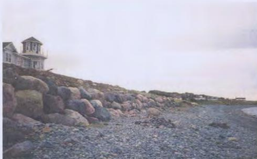
Plate 8.5: Boulder seawall constructed to halt erosion activity in segment 679 – 759 m. Note that the adjacent property is actively eroding and mitigation measures have not been put in place, potentially undermining the effectiveness of the seawall.
