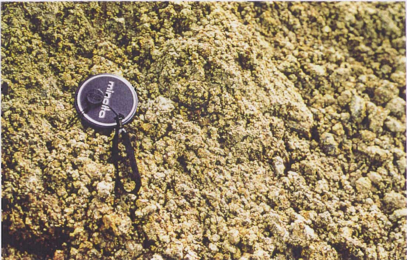
Photograph #2 - Test pit #2, close up showing soil characteristics
