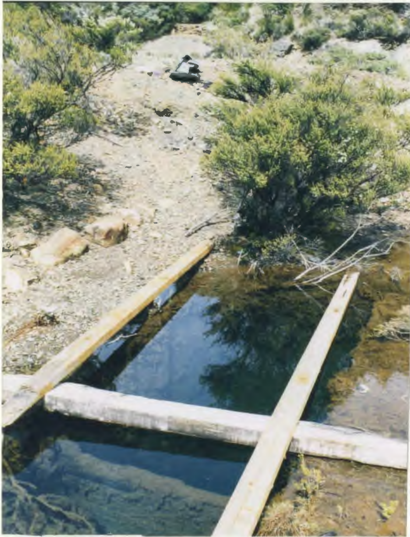
Plate 3.29 Abandoned shaft, east bank of Champion Creek, Champion Creek Mine (H-752). Wooden two-by-four beams mark shaft's entrance.
