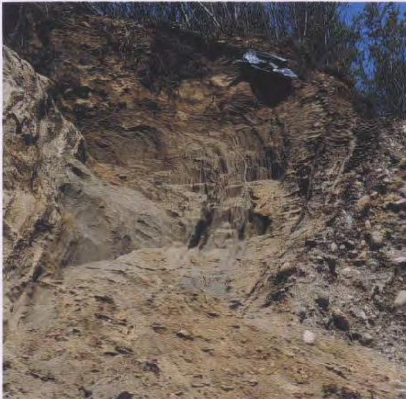
Plate 4-8: Steeply-dipping silt-clay within the upper part of the west face of Dawe's Pit. They were produced by loading from a rapidly sedimented sand bed that overlies the silt-clay.
