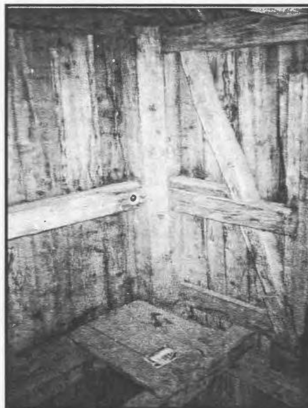
Figure 9 Second floor corner, interior, showing vertical posts, plate and diagonal bracing.
