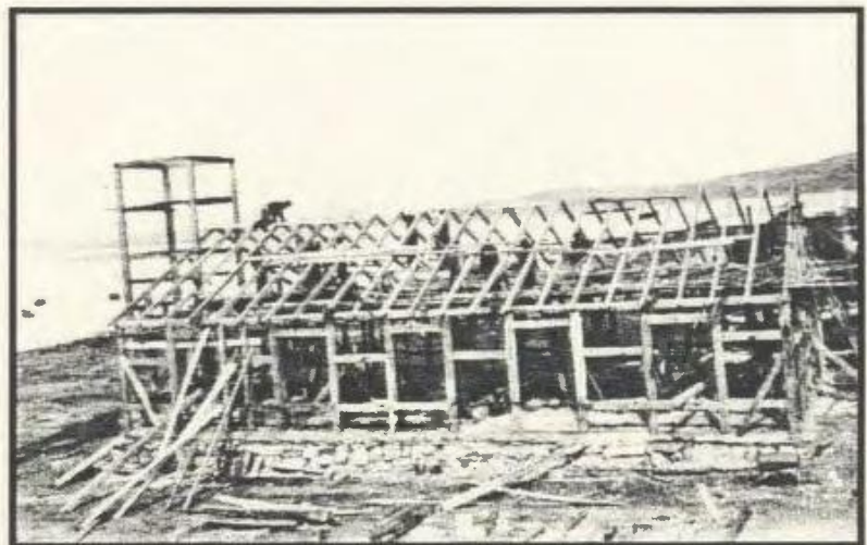
Figure 30 Nain church under construction, c1922, photo courtesy Moravian Museum, Nain.
