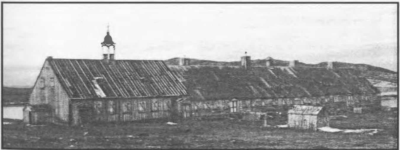
Figure 15 Hebron Mission complex, southern elevation.
