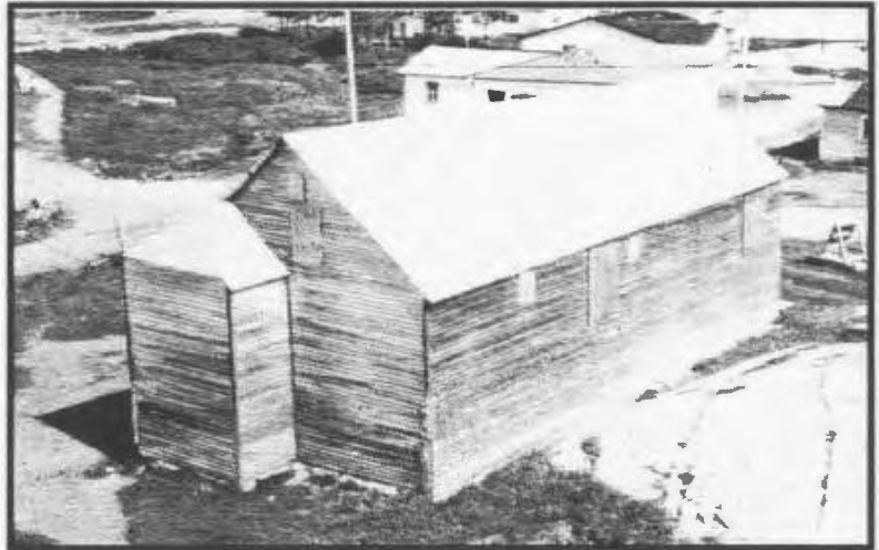
Figure 8 Rear view of 1782 Mission, showing addition on south side.
