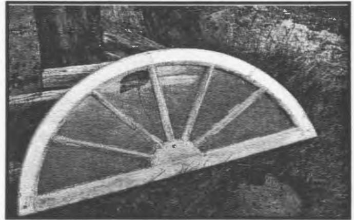
Figure 24 Georgian fanlight, removed from Hebron church portico.
