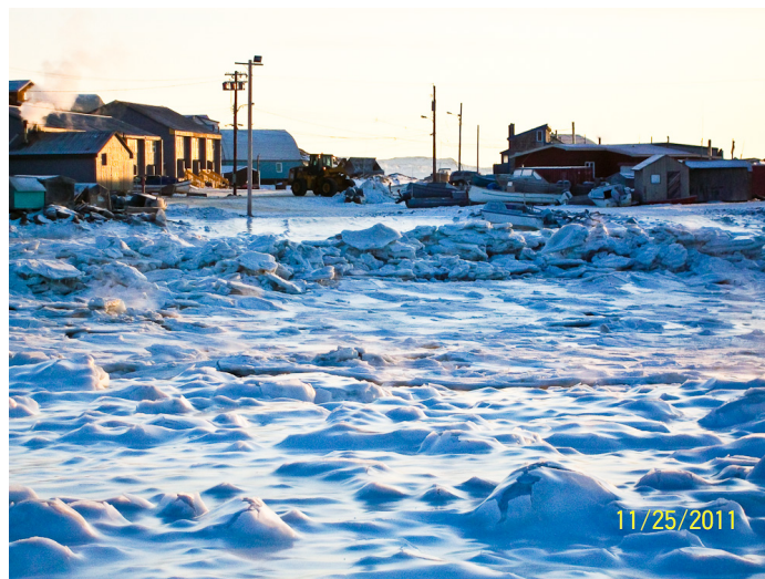
Figure 3.24: Light onshore winds with large ice floes in the nearshore produced ice pile-up on the boat ramp near the main breakwater in November 2011. A front end loader spent the morning clearing the debris off the ramp, which was piled roughly 2-3 m high.
