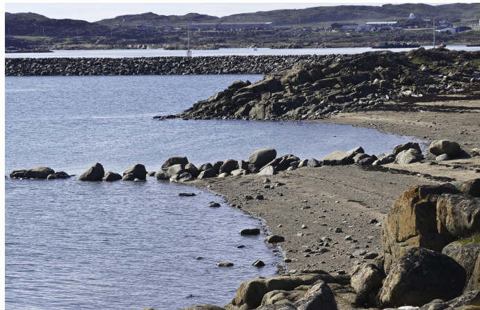
Figure 2.9: (photo SVH 2011-07-11) Pocket beaches created by both natural and artificial lateral confinement (outcrop at feet, groyne at far end of foreground beach, outcrop beyond, and breakwater/jetty beyond that). Photo taken at W end of cemetery beach (524501 m E, 706851 m N, facing WNW).
