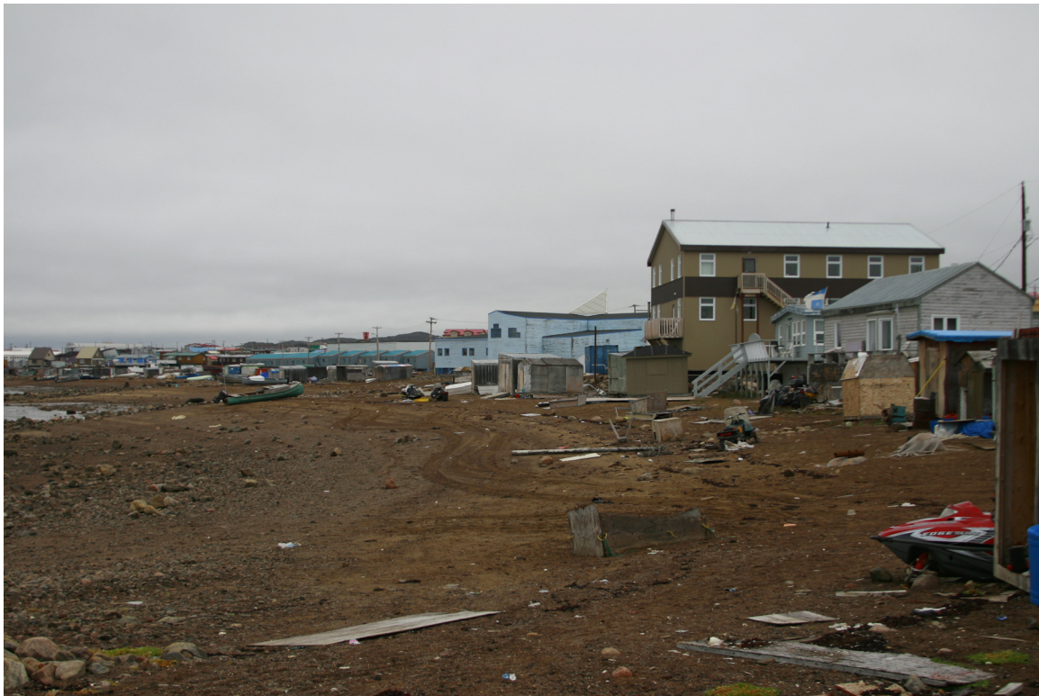
Figure 3.16: Coastal development on Iqaluit's shoreline. Note the lack of obvious backshore, with development on the beach face.
