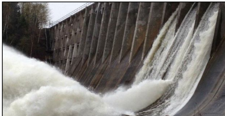
Figure 1.1: Deer Lake Power Opened Three Gates at a Main Dam on May 17, 2013
