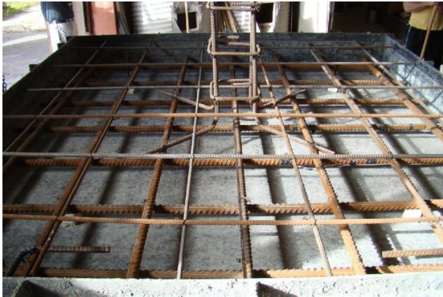
Figure 3.7. A reinforcement cage in the formwork for a typical slab
