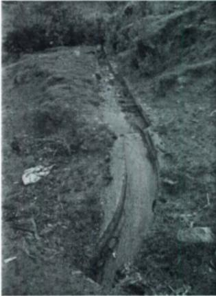
*Figure 4.4. Open-Lined Canal Flood Irrigation in Mullak'as-Misminay.*
