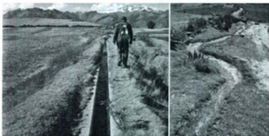
*Figure 4.9. Unpressurized lined and unlined irrigation canals in Mullak'as-Misminay.*
