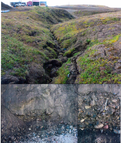
Figure 6.8 (above): Gully feature to west side of community. Note recent slumps in foreground caused by action of run-off and progressively deepening active layer, August 2008.
