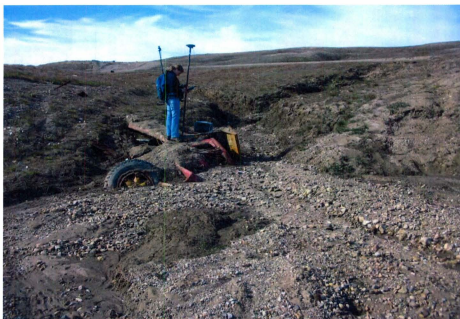
Figure 6.21: Recently resurfacing landfilled vehicle (c. 1980s) in west end gully, July 2005.
