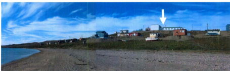
Figure 6.43: View of west side of Sachs Harbour from beach in July 2005. Note terraced character of development on this side of community. Concerns are being expressed about ground conditions in the vicinity of the steep bank below the school (see arrow).
