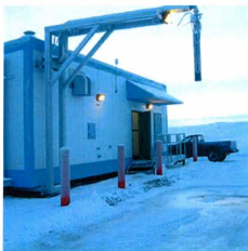
Figure 6.24: Truck fill station at water treatment plant, Sachs Harbour. (Photo: MACA)
