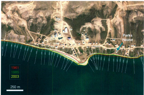
Figure 6.11: Sachs Harbour shoreline change 1961-2003. While the community beach has grown, retreating bluffs to the east and west are encroaching on residential infrastructure. Source: Natural Resources Canada courtesy G.K. Manson (data). Contains material © DigitalGlobe. Figure © Her Majesty the Queen in right of Canada, 2005, with permission.
