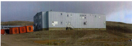
Figure 6.41: Ikaahuk Co-operative Building, August 2008.
