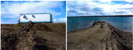
Figures 6.23: Sachs Harbour Water plant (left) and intake (right), July 2005
