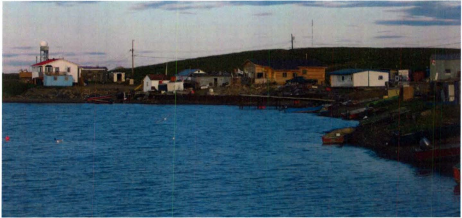
Figure 5.22: Property armoring on Inner Harbour-side of community, August 2006
