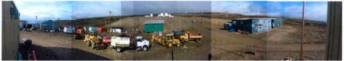
Figure 6.22: Panorama shot from Hamlet garage looking north. Power plant to left; tank farm up hill; and shared Hamlet/Parks Canada Interpretation Centre building to right (arena visible to rear). A buried fuel line follows the road from the tank farm down the hill to the beach. August 2008.
