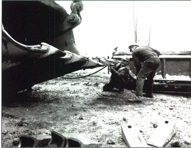
Figure 11. Two men, including Innu labourer Augustin Vollant, are busy changing a tooth on a Marion shovel bucket, Redmond mine, December 1969.
