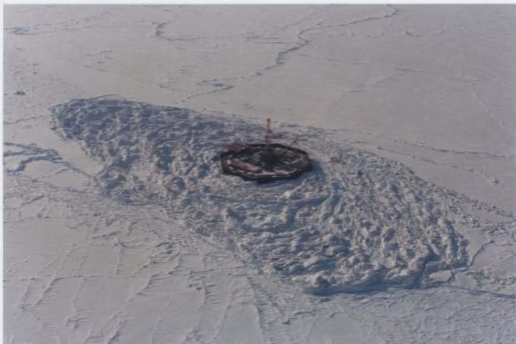
Aerial view of Caisson Retained Island (CRI) at Kaubvik, May 1987.
