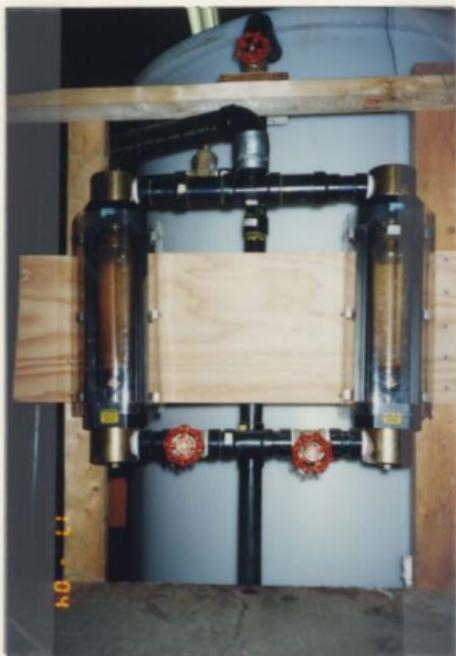
Figure 3.3. Photograph of the flowmeters model # 10A3555A
