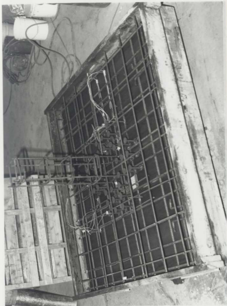
Figure 4.10: Shear-stud reinforcement (Studrail) in construction (Slab HS22)
