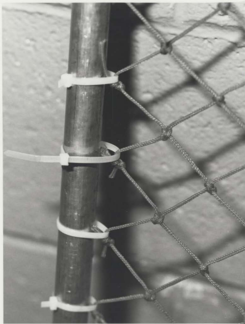
Figure 3-3 : Electrical cable wraps used to attach nets to frame
