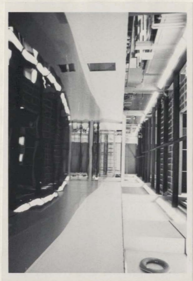
FIG. 3. REGULAR WAVE IN WAVE TANK
