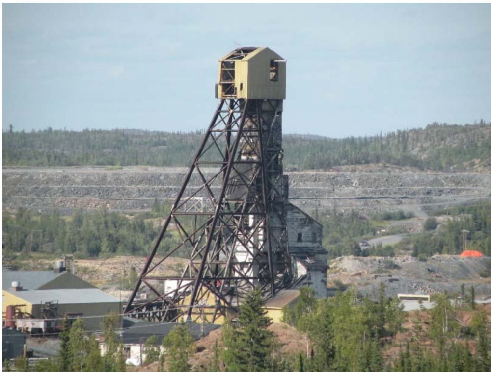
Abandoned headframe, Giant Mine. Photo by John Sandlos and Arn Keeling.
