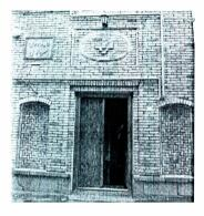
Figure 130: Sattarkhan house, blind windows, a courtyard wall containing the brickwork in forms similar to windows. Such forms may be used by people to compensate for the lack of other decorations in the facade.
