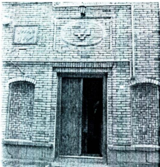
Figure 130: Sattarkhan house, blind windows, a courtyard wall containing the brickwork in forms similar to windows. Such forms may be used by people to compensate for the lack of other decorations in the façade.
