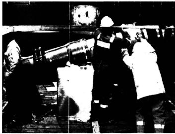
Figure 3-11: Fitting anodes on flexible pipe (SUT, 2002)
