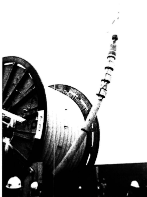
Figure 3-10: Maneuvering end of flexible pipe with ROV hook (Technip, 2011)
