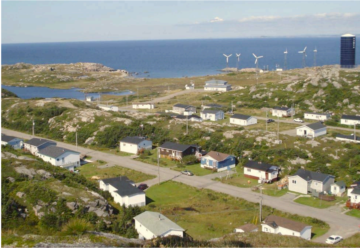
Figure 2: A view of Ramea showing six, 65kW wind turbines and community water tank.
