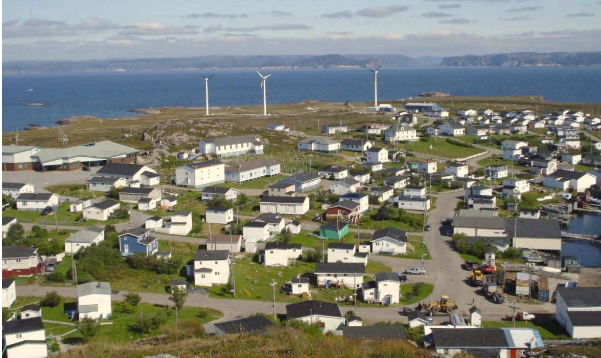
Figure 1: A view of Ramea showing the community, diesel plant and three recently installed 100kW wind turbines
