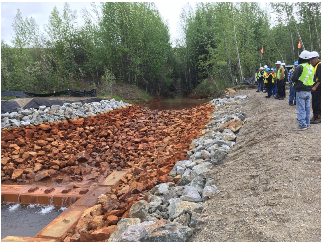
Figure 6.2 Elders Inspecting the X13 sump, located in the Down Valley area (down river from the Cross Valley Dam), a low area where water seeping under the dams is collected and pumped back for treatment. Caitlynn Beckett, Elders tour of the Faro Mine Site, June 2019.
