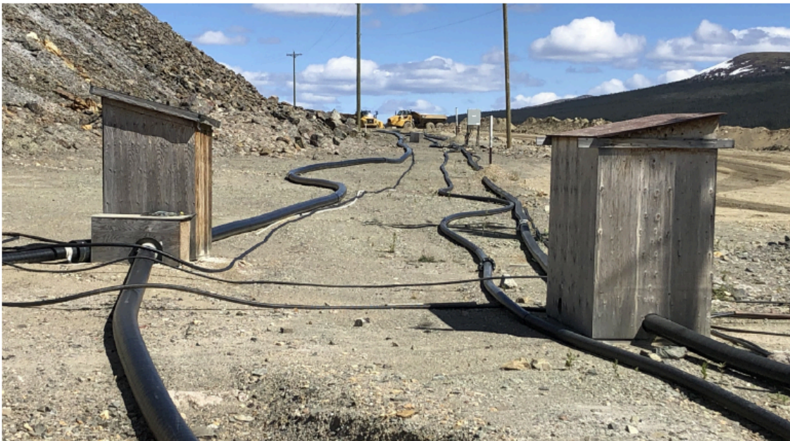
Figure 6.1 Components of a groundwater collection system that transports contaminated water that originates in waste rock to the Faro Pit, where it will be temporarily stored before treatment at the water treatment plant. Photo taken from: Faro Mine Remediation Project, “Plain Language Summary,” submitted to YESAB (August 2021). YESAB Registry 2019-0149-0638.
