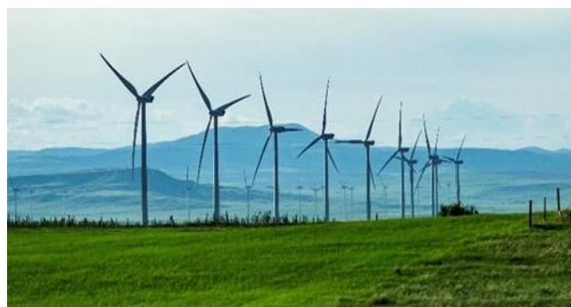
Figure 1: Wind Power Plant [7]
