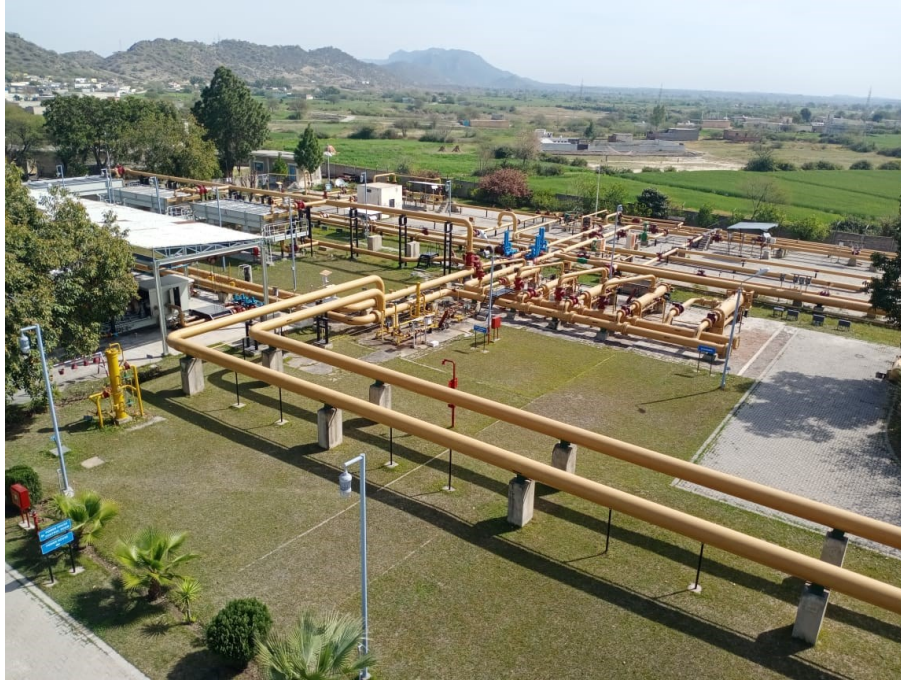
Figure 2.2. Actual view of selected site
