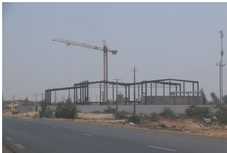
Figure 4: Barna plant in construction (Kayar, Senegal) (source: Olivier Randin).
