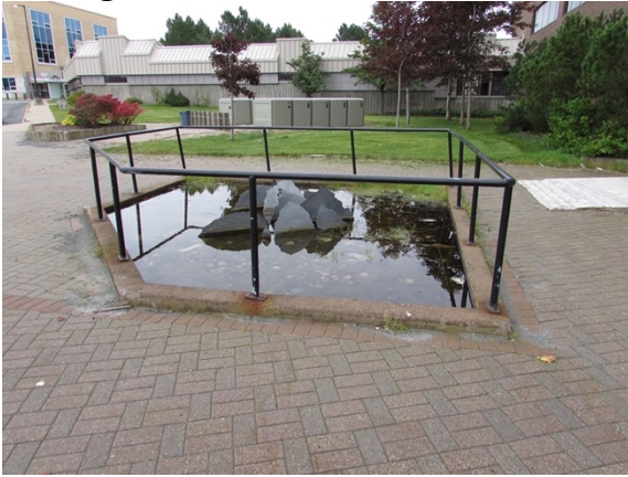
Figure A54 Image of the Icebergs Monument outside of the Confederation Building. Emlyn Tuck (2023).
