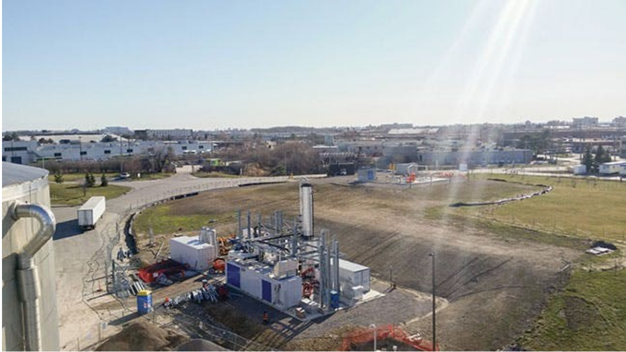
Figure 5. Dufferin Organics Processing Facility in Ontario (Source: Biogas Community, 2023)
