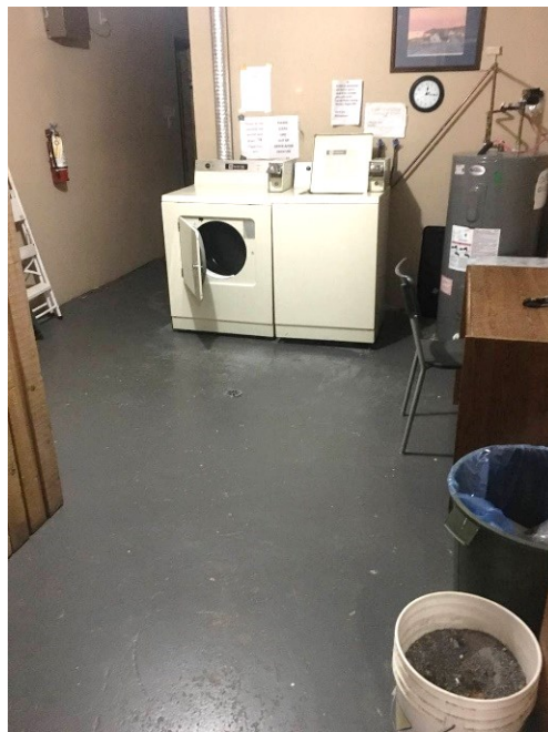
Figure 5.17: Shared Laundry Space, Corner Brook
