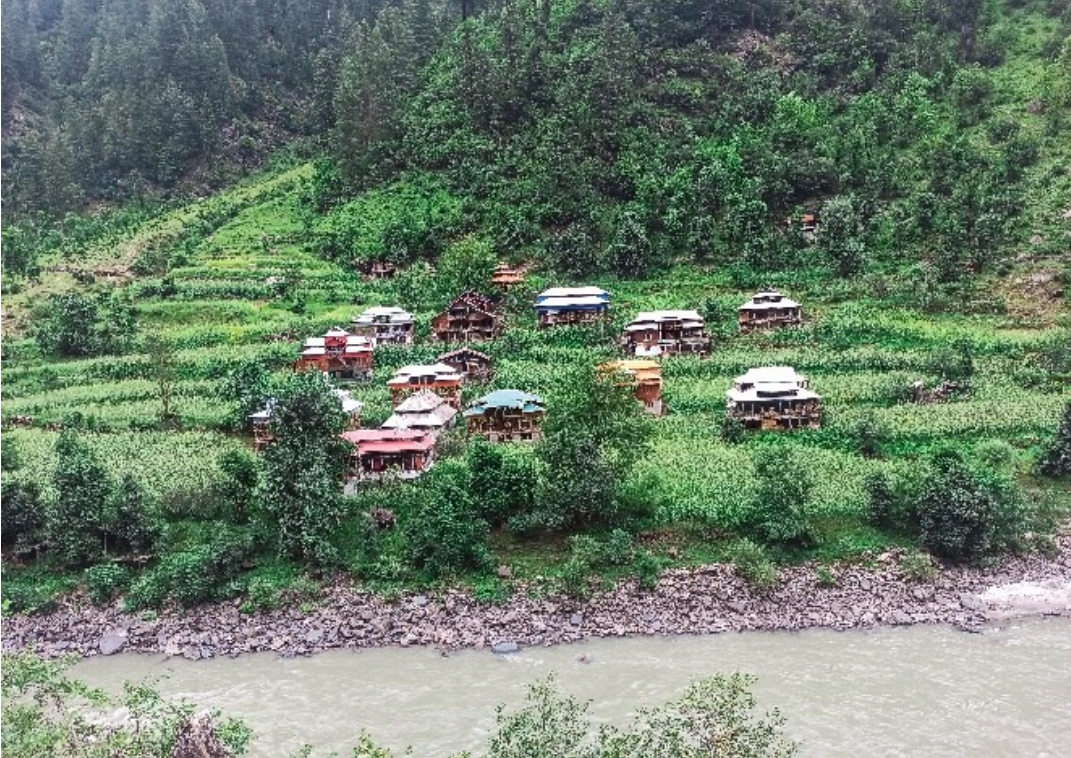
Figure 2.2. Aerial view of the proposed site
