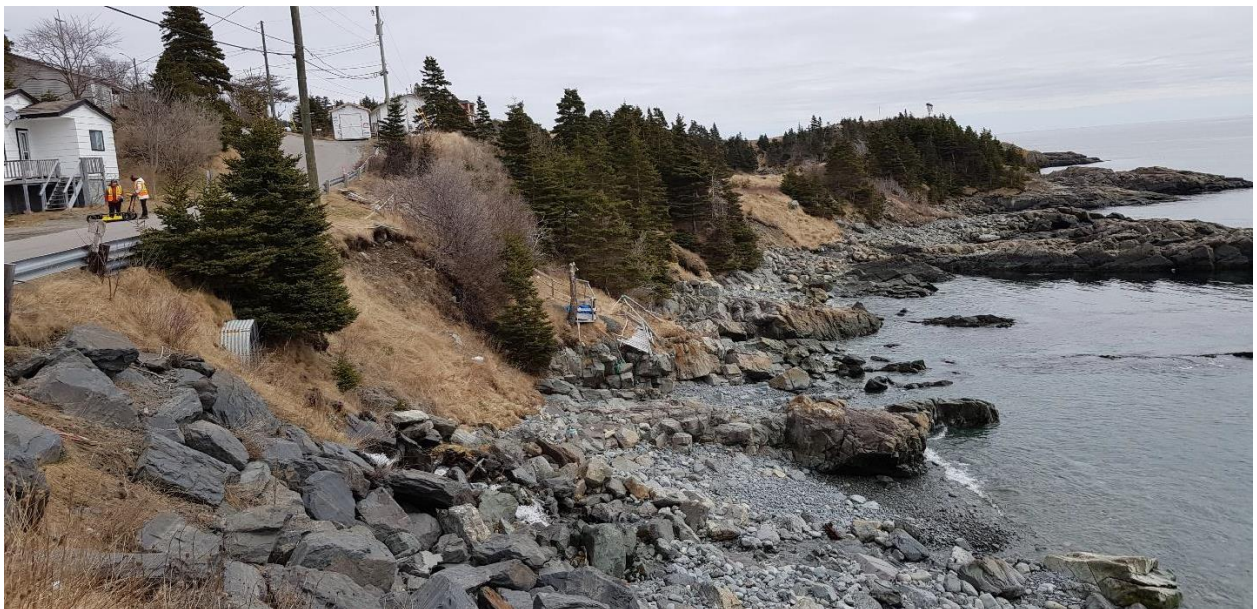
Figure 2-3) View of the beach at the Bread and Cheese site, looking east. Rip-rap and the bay end of the culvert are seen to the left. (1 April 2021).
