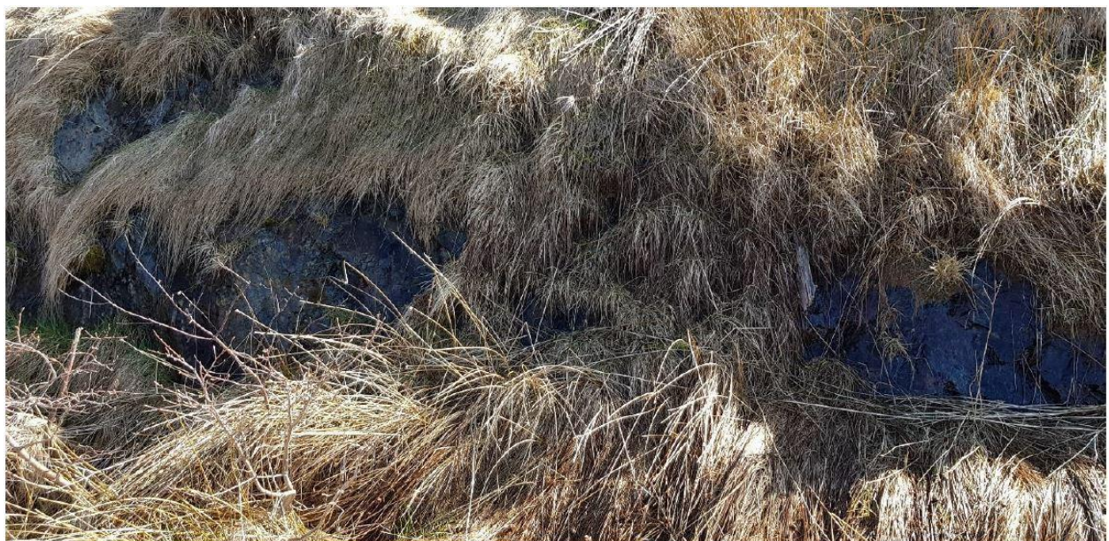
Figure 2-21) Bedrock showing underneath vegetative cover on the slope above Northside Road, Cliff site, a few metres southeast of the deck shown in Figure 2-20.
