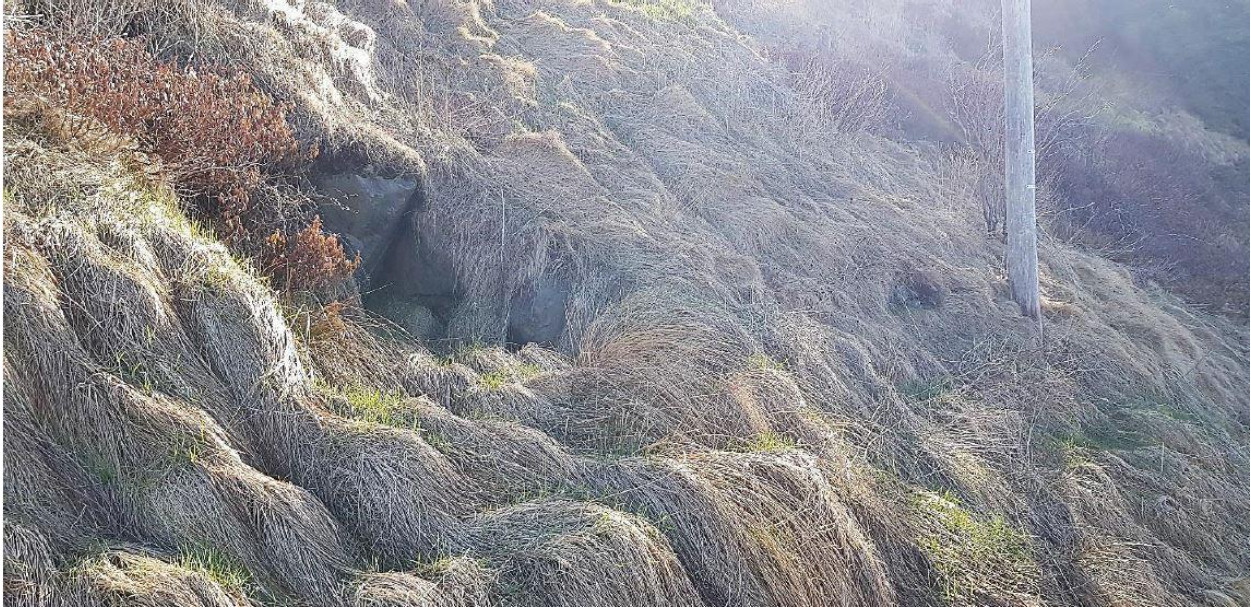
Figure 2-22) Creeping of surficial turf, with some accumulation behind the street light pole seen on the right in Figure 2-20. Some boulders are seen within the grassy slope.
