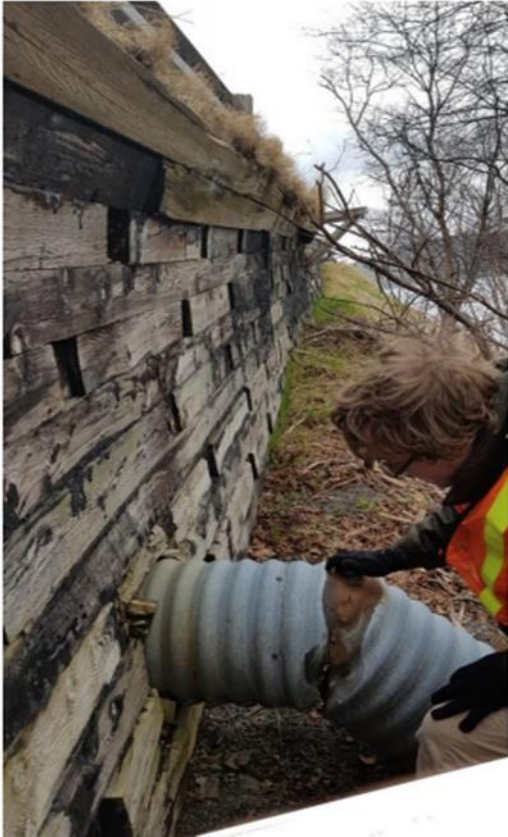
Figure 2-17) side view of the wall near culvert 1.
