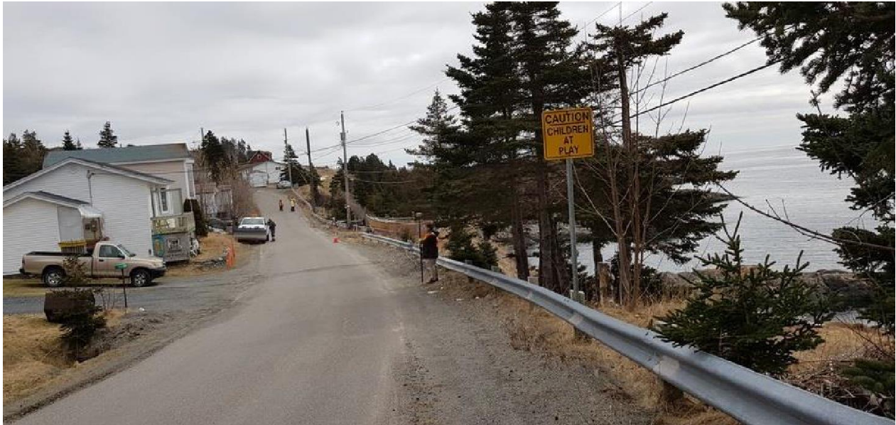
Figure 2-2) Gunridge Road, looking east. Field assistant Jason Sylvester is holding the RTK rover near the west end of the GPR survey grid. (1 April 2021).
