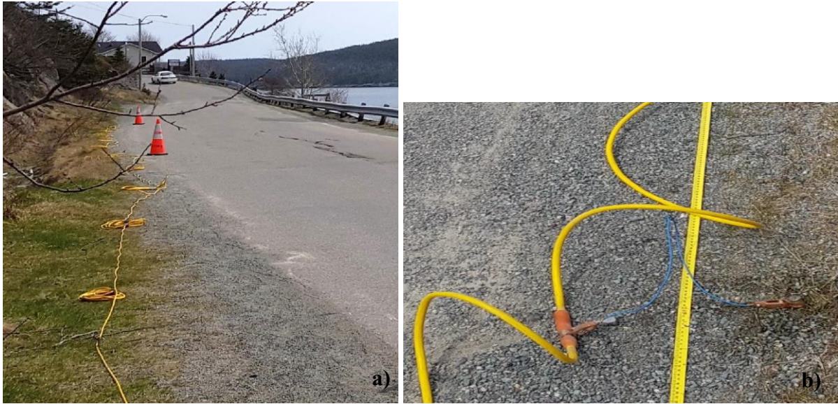
Figure 4-3) a) DCR multicore cable spread out along the road side. b) DCR multicore cable showing take out (orange) and a blue wire with bulldog clips each end, connecting callout to the top of a steel electrode (white arrow) hammered into the ground. The Cliff site, 26 April 2021.
