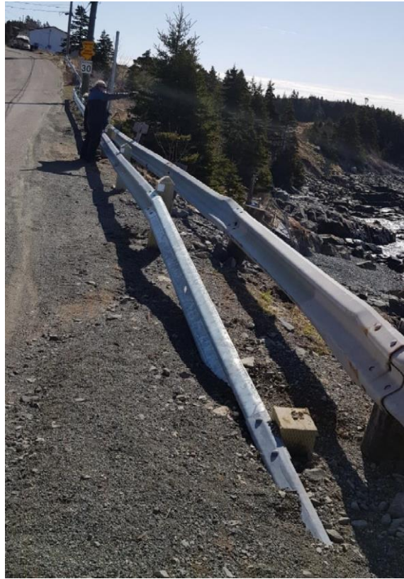
Figure 2-13) New railing constructed inside older railing. Looking east, Bread & Cheese, 21 April 2022.
