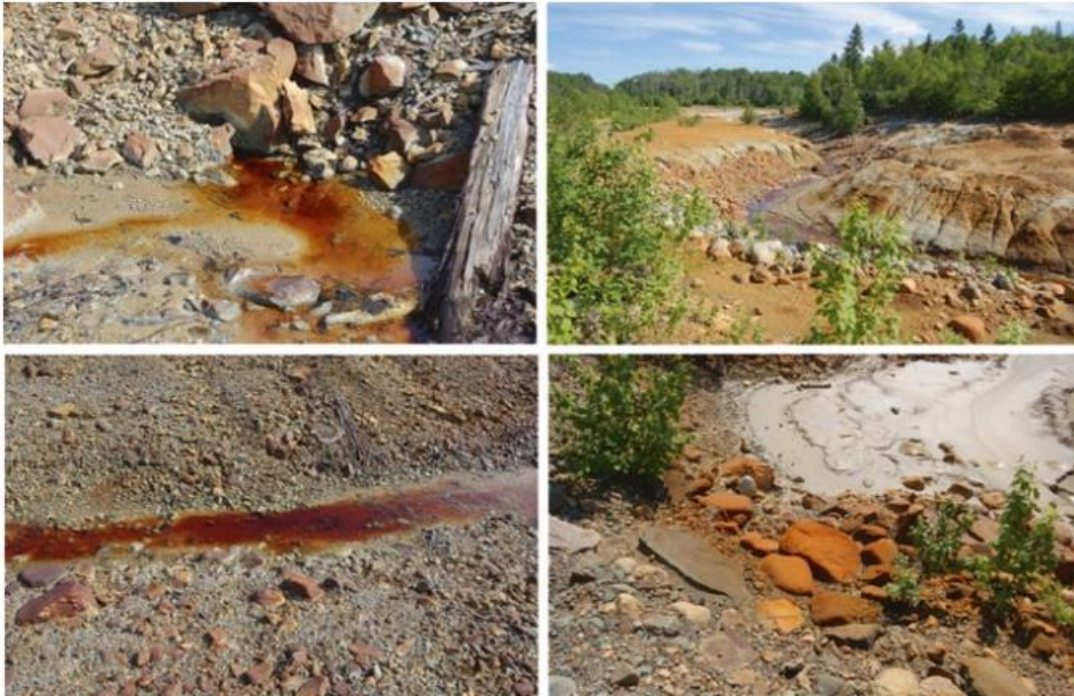
Figure 2-23: The formation of acid mine drainage as a result of mineral processing (Yilmaz et al., 2017)
