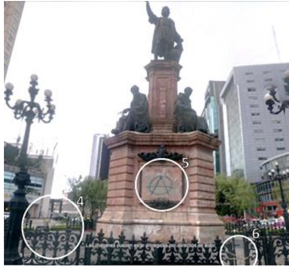
Figure 43. The sculptural complex's deterioration and graffiti. Source: Daniel Morales (2016).
