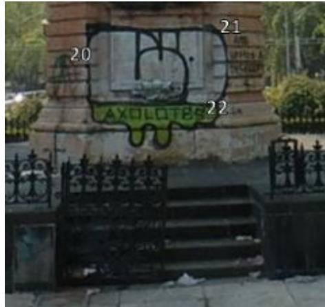
Figure 50. December 2018, we can observe more graffiti and trash on the monument's steps. Source: Israel C.
