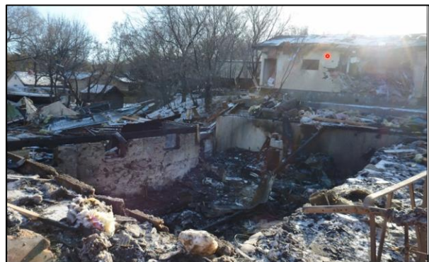
Figure 1.1: Explosion in December 2014 in Saskatchewan due to leaking of gas distribution pipe (CBC 2014)
