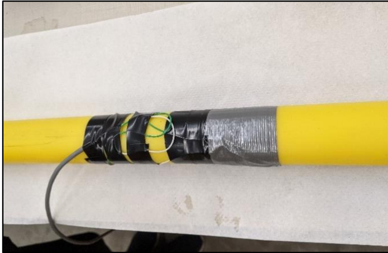
Figure 5.7: Strain gauge installation including electrical wires and protecting wraps
