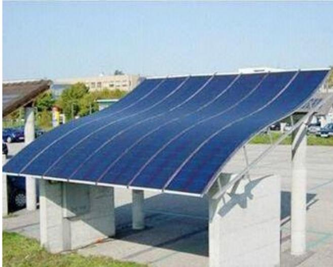
Figure 4: Thin Film Panel [13]
