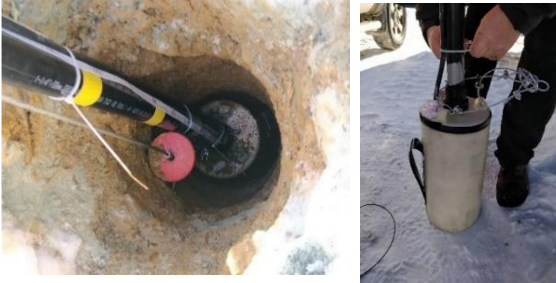
Figure 5-4 Downhole survey with GPR unit protected
