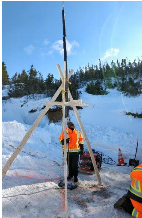
Figure 3-1 Wood shelf for the GPR cable hoisting
