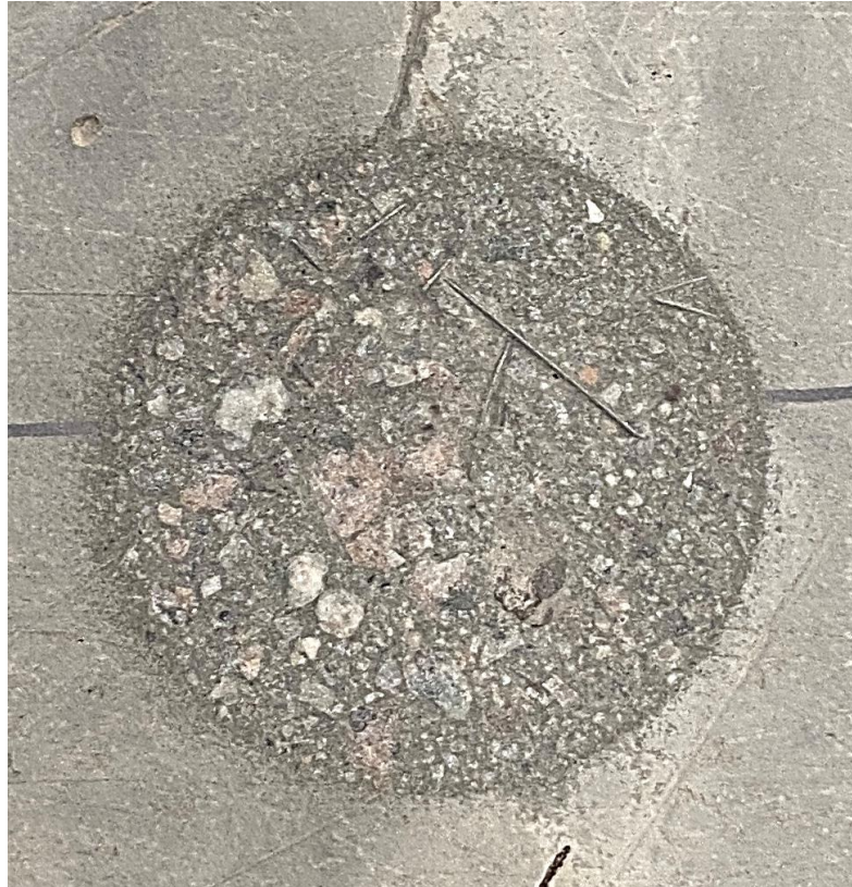
Fig. 4-20 CCSFs specimen tested area sandblasting method.
