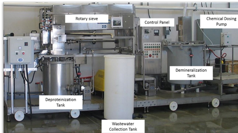
Figure 1. 19 Chitin pilot processing line (Photo Courtesy of CASD, Marine Institute, MUN)
